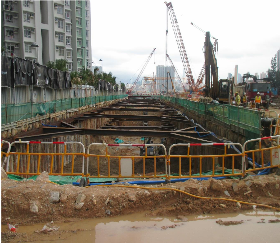
Pipe Pile Wall
